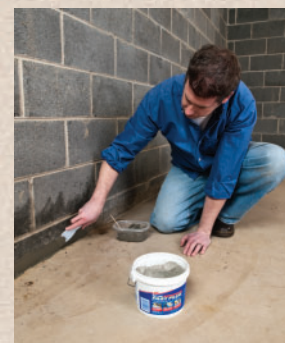
Patch all holes and cracks with DRYLOK Fast Plug.
