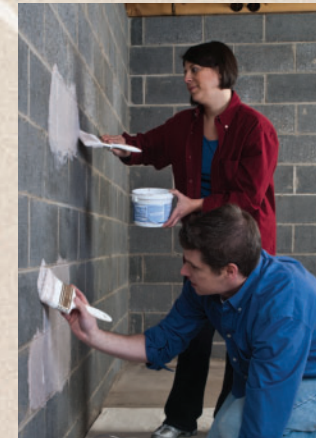
Apply DESIGNER DRYLOK with a good quality nylon bristle brush.
