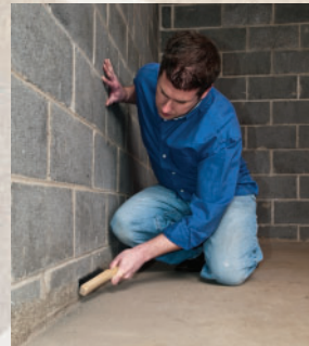
Clean masonry surfaces thoroughly with a wire brush.
