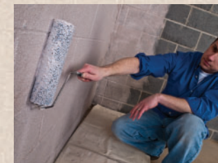
Apply the second coat.
