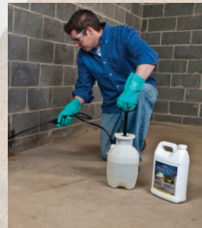
Clean efflorescence with an etch solution.
